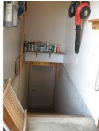
door from garage to basement
